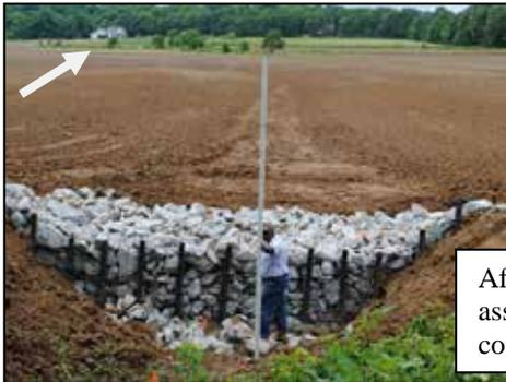
After: The farmer, with our technical assistance, installed a drop structure to control the head cut.
