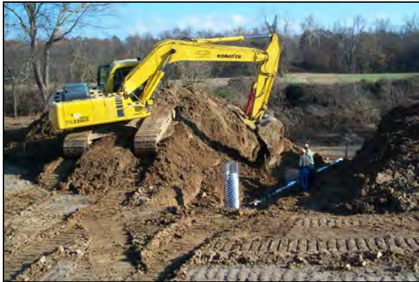
Among other practices seven Grade control were installed through TDA grant funding, 2 along the banks of Turkey Ck, a 303d stream
